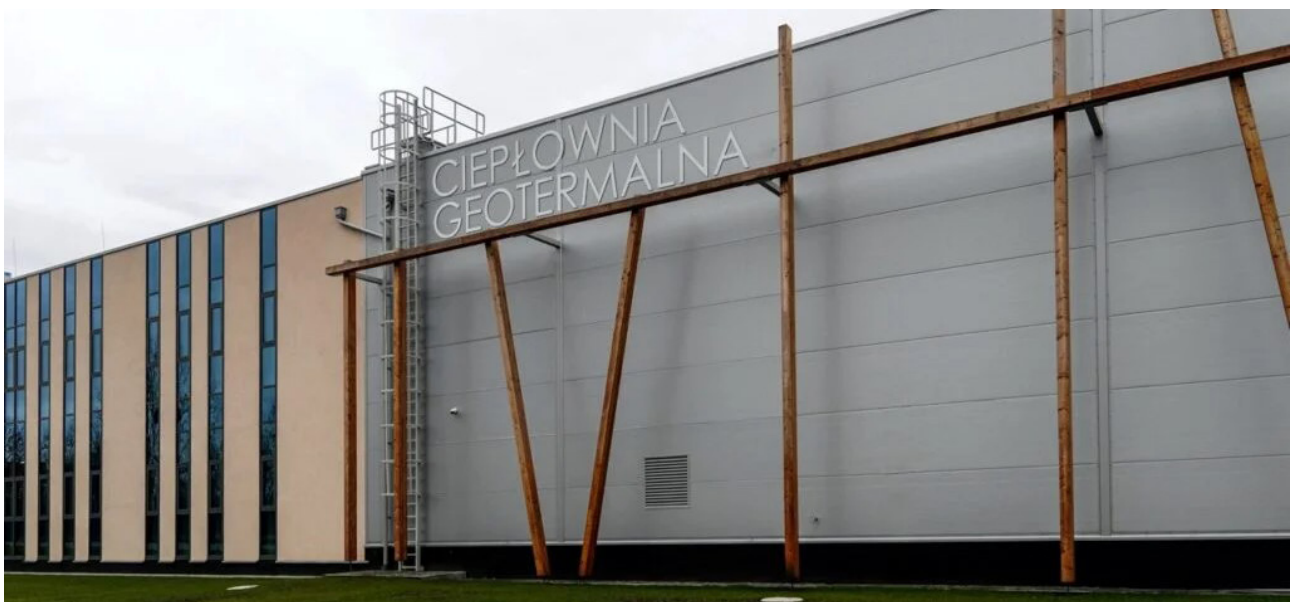
Geothermal heating plant in Konin, Poland (source: Geotermia2030.pl)
